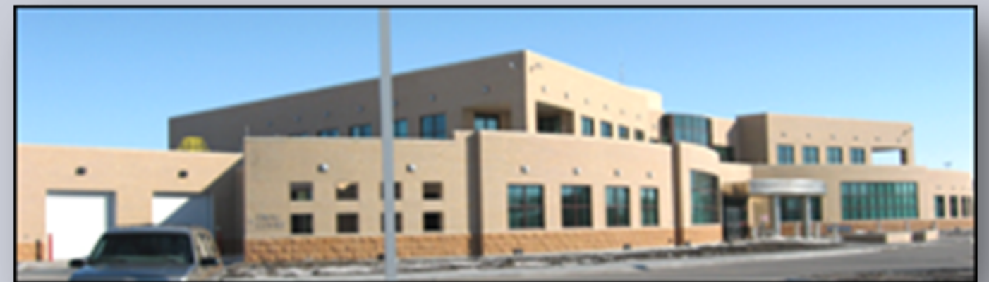
Grand Island - Hall County Law Enforcement Center, completed in 2008
