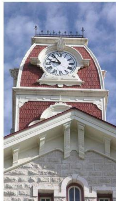
Sheet metal roofing at tower, Parker County Courthouse
